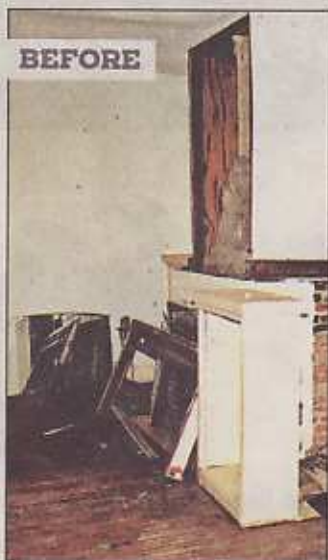
The Kimballs' fireplace renovation: In the beginning, BEAU KIMBALL
